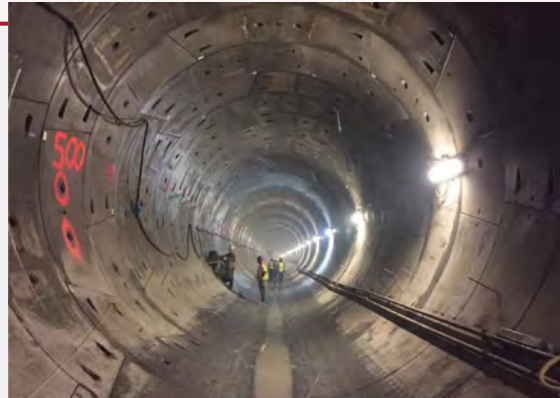
First Street Tunnel (Source: DC Water, No Date)
